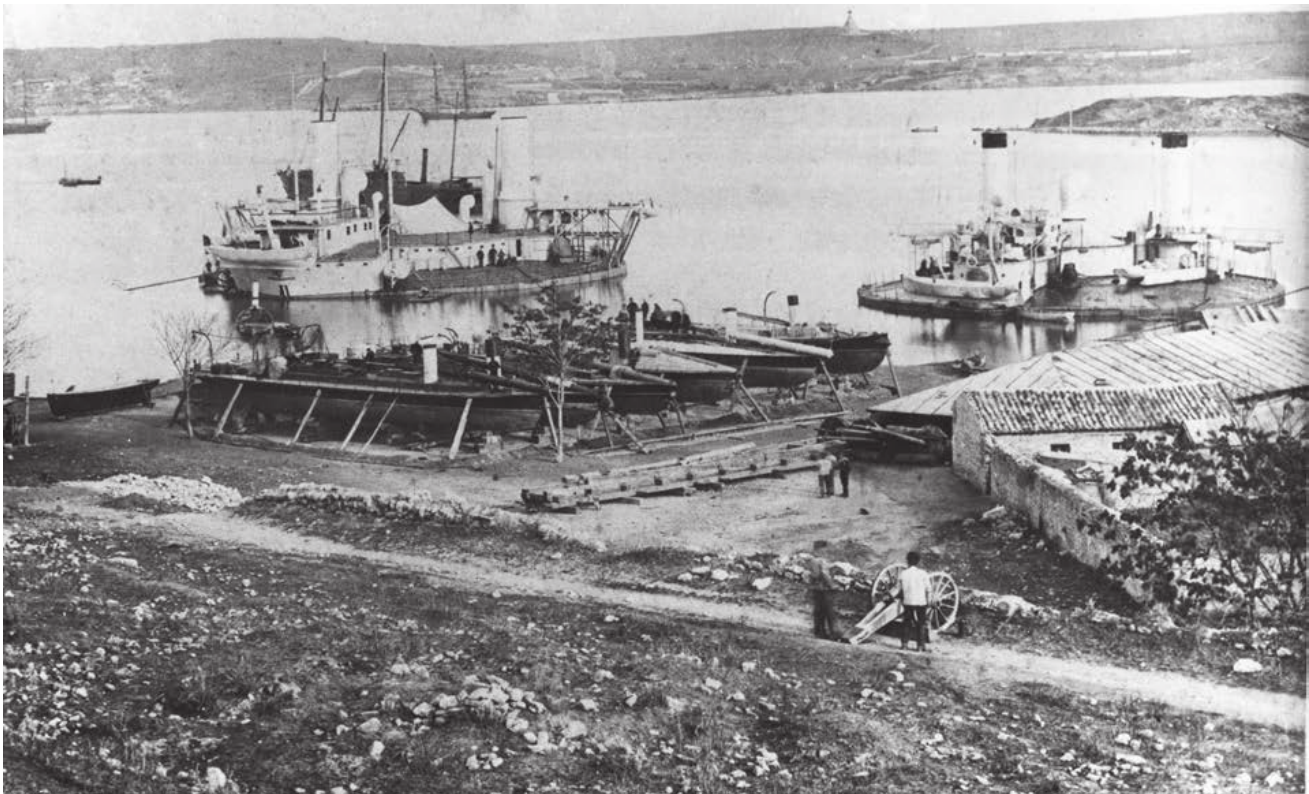
Vitse-Admiral Popov (left) and Novgorod (right) in Sevastopol's Southern Bay (Iuzhaia buхта) in the 1880s. Note the six small torpedo boats hauled up on shore; these appear to be several different types of first-generation boats, built at the time of the Russo-Turkish War of 1877-78; originally equipped with spar torpedoes, these craft were rearmed with tubes for Whitehead torpedoes in the 1880s. (Courtesy of Sergei Vinogradov)
