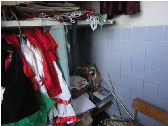
Picture#30: Old bathroom converted into storage room
