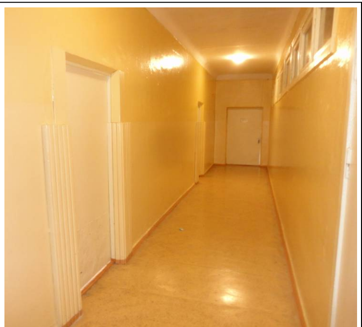
Picture#73: Gymnasium Hallway. Replace doors to the locker rooms and restore all conditions as they were before the door replacement.
