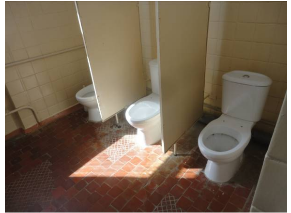
Picture#35: Typical girls' toilets in West Wing. All to be replaced with new.
