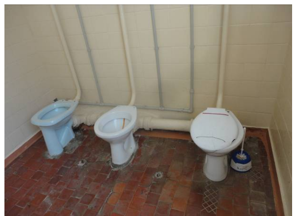
Picture#33: Condition of existing bathrooms
